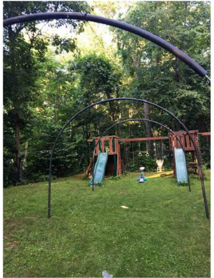
Figure 4 - The arches inserted into the ground stakes
